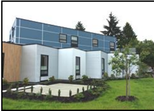
Foundry Comox Valley
